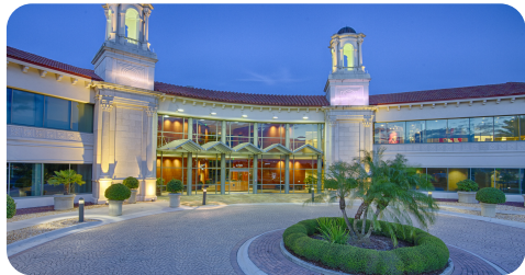
Outside View of Building
